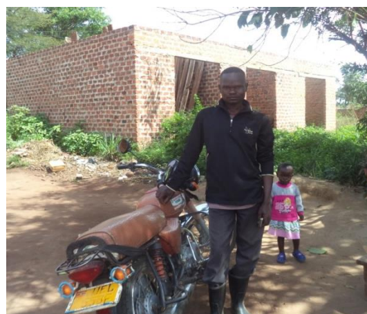
Mr. Magezi Isma has started constructing an improved house using a loan from SHUF.
