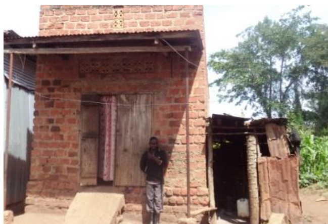
Mr. Magezi Isma of Kikube scheme in Luwero Sub-county, Luwero district front of his old house.
