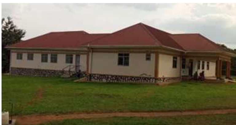
A side view of the health centre complex
